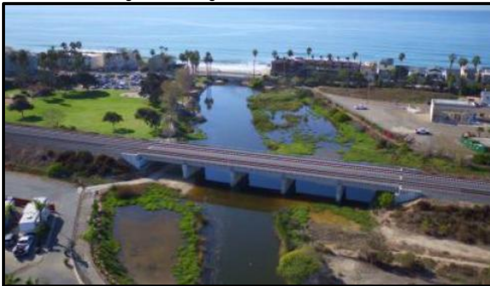
Figure 3: Bridge over Loma Alta Creek
