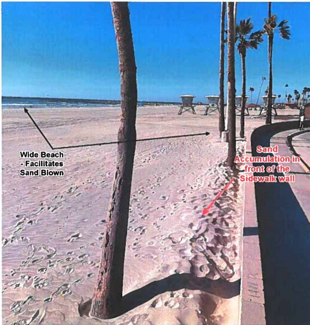
Figure 3. Sand accumulation west of the sidewalk wall at Harbor Beach, and wideness of the beach.
