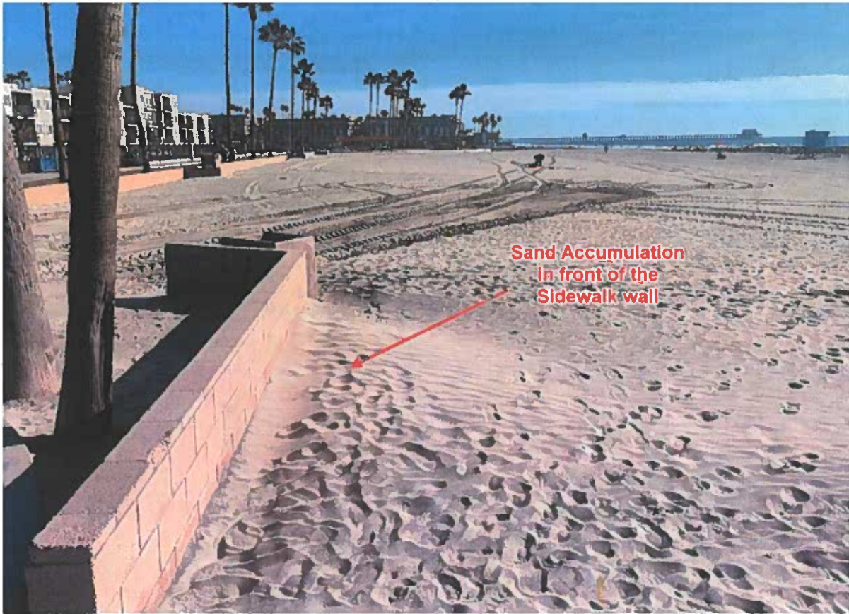
Figure 2. Sand accumulation west of the sidewalk wall at Harbor Beach.
