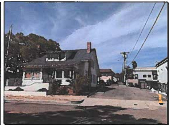
VIEW FROM CLEMENTINE ST LOOKING EAST UP ALLEY. SUBJECT PROPERTY ON LEFT
