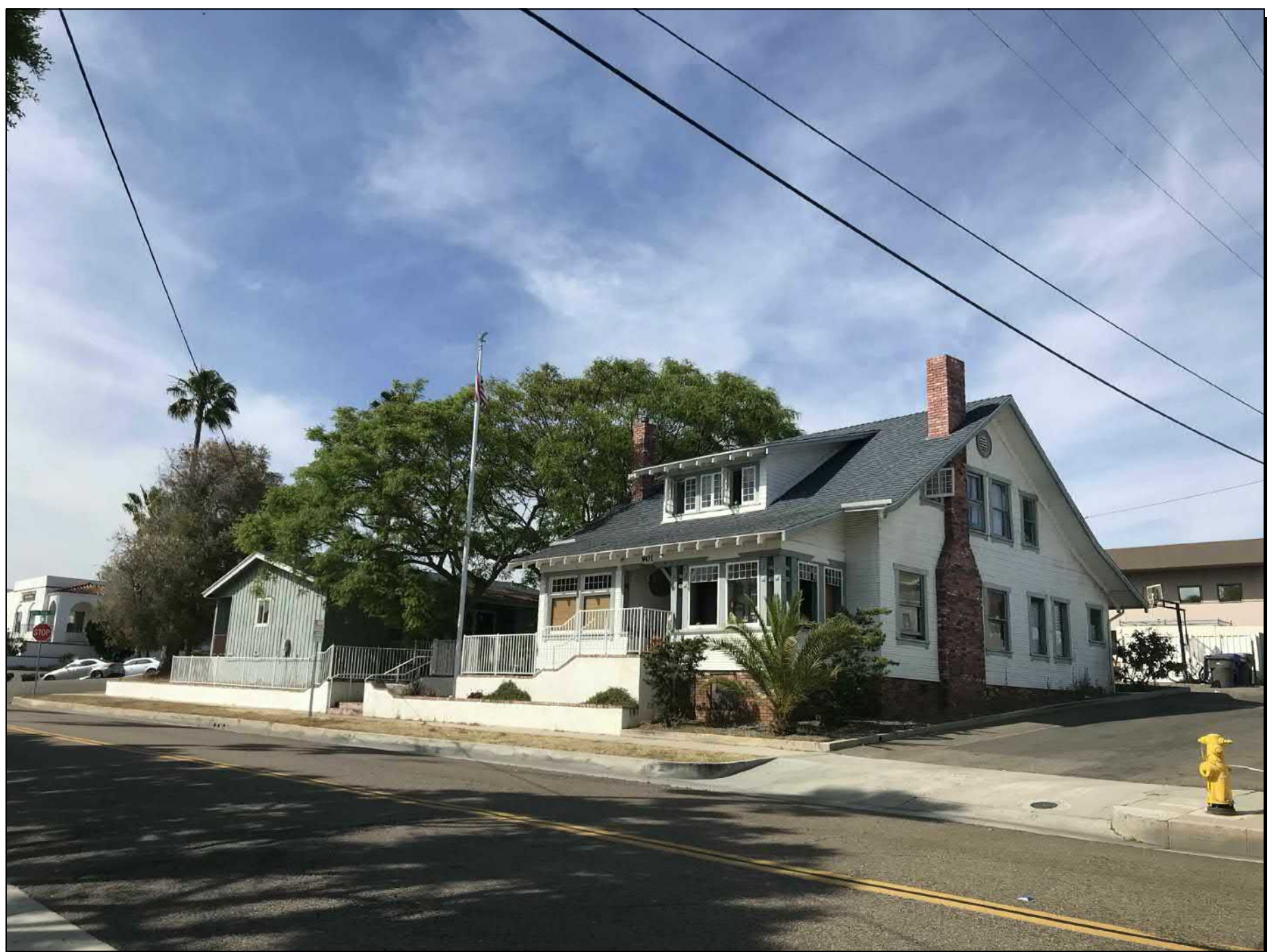
VIEW FROM CLEMENTINE ST LOOKING NORTH EAST AT SUBJECT PROPERTY
